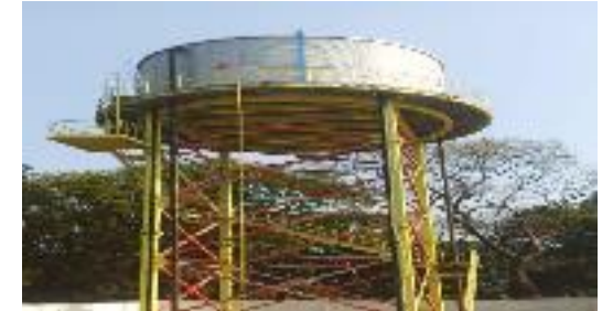
Water Tank, Uttar Pradesh
